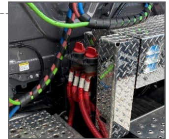
Figure 13. Driver-side battery disconnects
