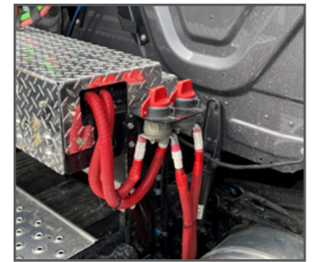
Figure 12. Passenger-side battery disconnects
